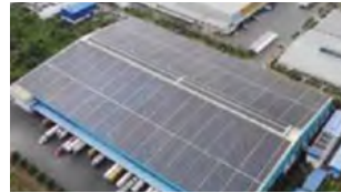
Installation of solar panels at CJ Gemadep Refrigeration Logistics Center
